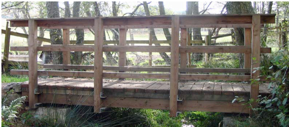
Fig. 2 – Example of 7m footbridge
